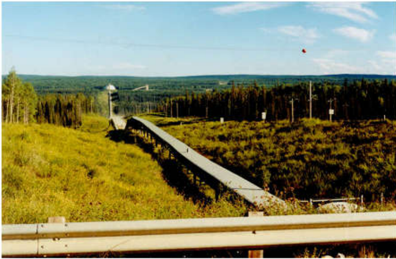
From Emerson Creek Road, looking southeast, toward the Athabasca River, CN railhead and Highway 16.
