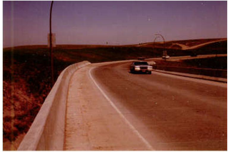
Former Deerfoot Trail SB on-ramp (which has been replaced by a much longer loop), looking northeast. 16
