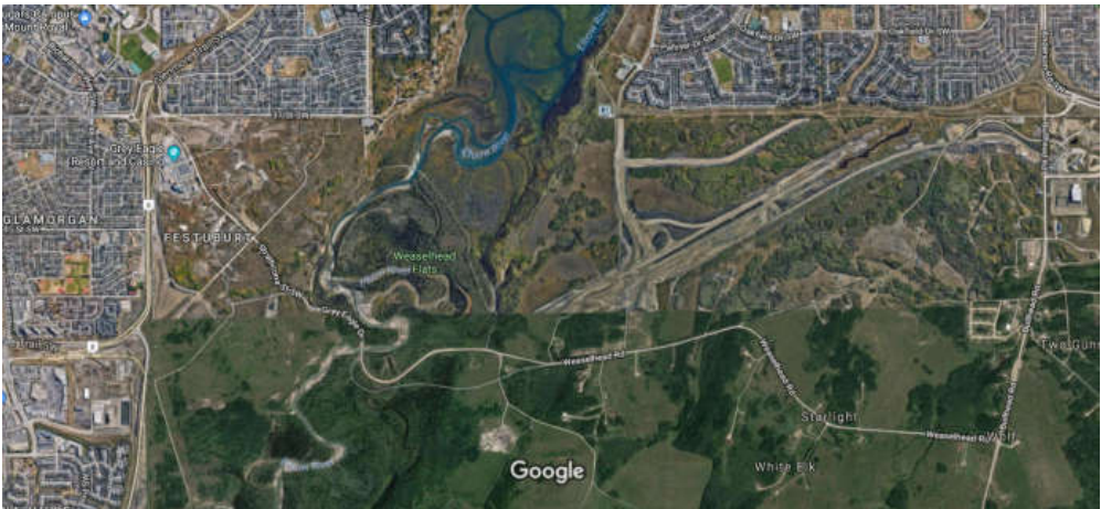
Something under construction through the Weaselhead.
