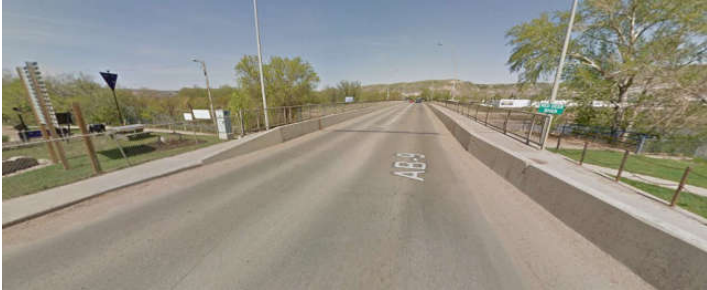
Red Deer River Bridge, Drumheller, 2019.
