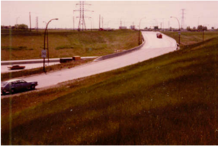
Deerfoot Trail SB off-ramp to Peigan Trail, approaching an overpass; looking southeast; this ramp remains in use.
