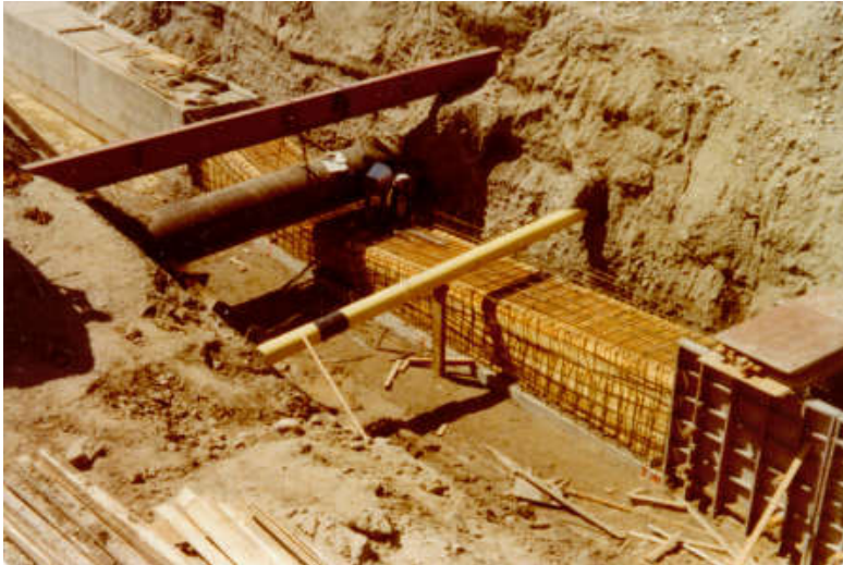
Concrete box culvert transition section, looking southwest, and note that the watermain is suspended by a beam.
